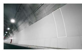
3plus, 5plus and 6plus laminated porcelain stoneware can be laid on curved surfaces, both concave and convex. Products with particular finishes can have certain limitations depending on the geometry of the slab, so please contact the Panariagroup Technical Department before proceeding with the installation.
