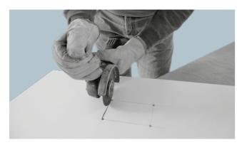
To obtain internal and L-shaped corners, round off the vertices of the internal corner using drill bits with a diameter of at least 5 mm to reduce the risk of breakage.
