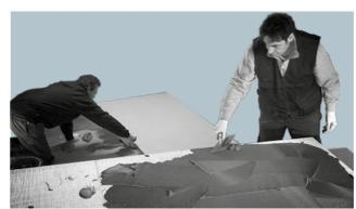
Apply adhesive on the substrate and on the back of the slab by spreading the adhesive full-bed over the entire surface to be covered, using a notched trowel with tilted teeth that are spaced 6 mm apart (e.g. Raimondi art.184HFV6) Then apply the adhesive also to the rear of the slab using a 3 mm square notched trowel. When installing on floors, remember to spread extra adhesive around the edge of the slab.
