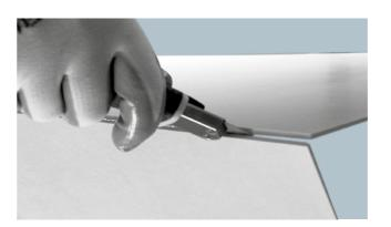
For 3plus, 5plus and 6plus laminated porcelain stoneware, after scoring the ceramic part and splitting the slab, complete the operation by cutting the fibreglass mesh with a standard
