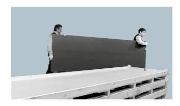
When the slab is upright, hold it from its top edge and shift it keeping it straight and upright. This operation should be performed with the aid of a second person.
